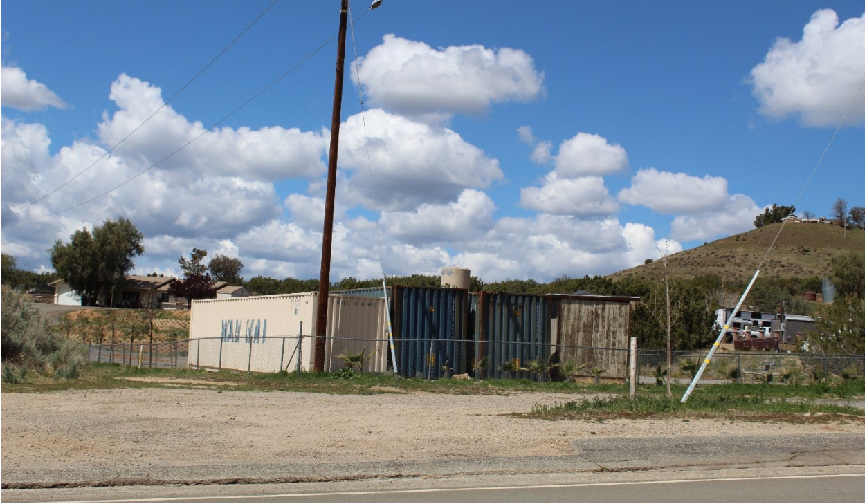
Illegal Commercial Outdoor Storage Use in an Agricultural Zone.
