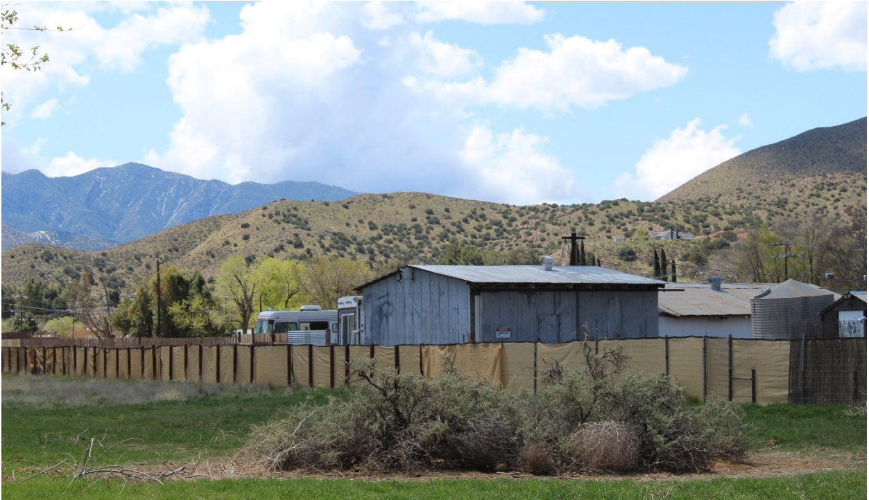
Illegal Commercial Outdoor Storage Business in a Residential Zone.
